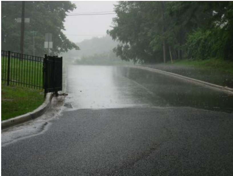
Pervious asphalt at Willard Beach Park
