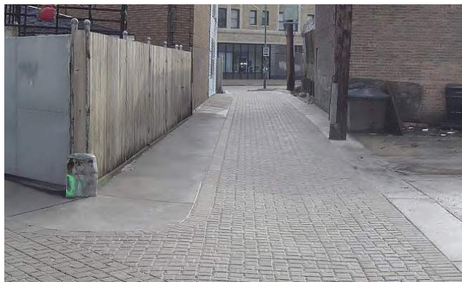
(Above) Permeable block alley after reconstruction and (right) before reconstruction.
