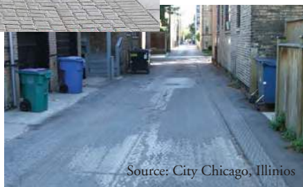
(Above) Permeable block alley after reconstruction and (right) before reconstruction.
