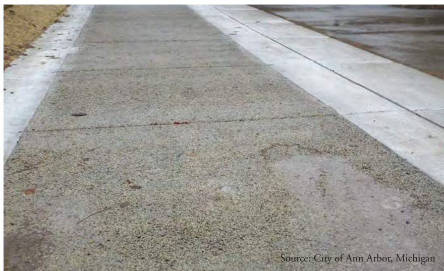
Completed permeable concrete alley.
