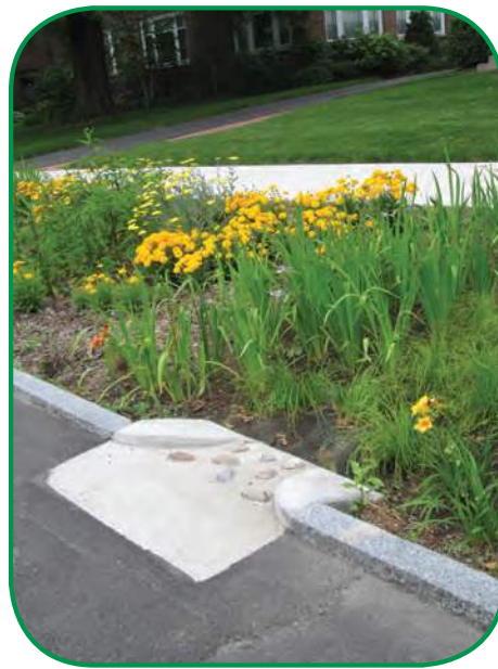
Energy dissipater between road and bioretention.
