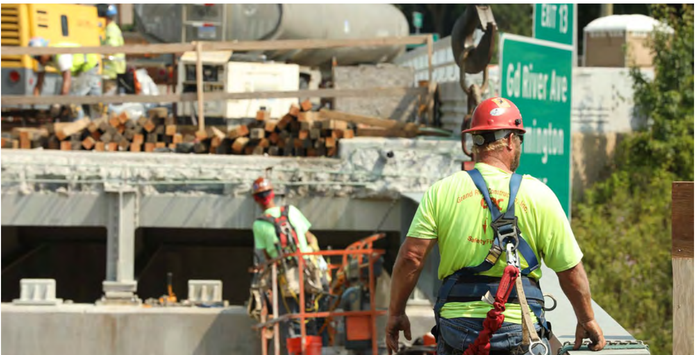
GRAND RIVER AVENUE (M-5) CONSTRUCTION
