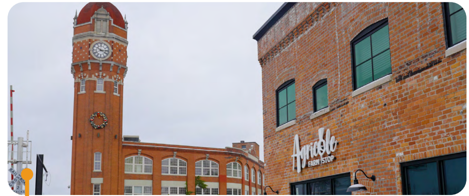
Once a water tower, the clocktower in downtown Chelsea has been used for many other purposes, including as a wedding venue and for offices. The building is also an icon, often used in logos and photos.
