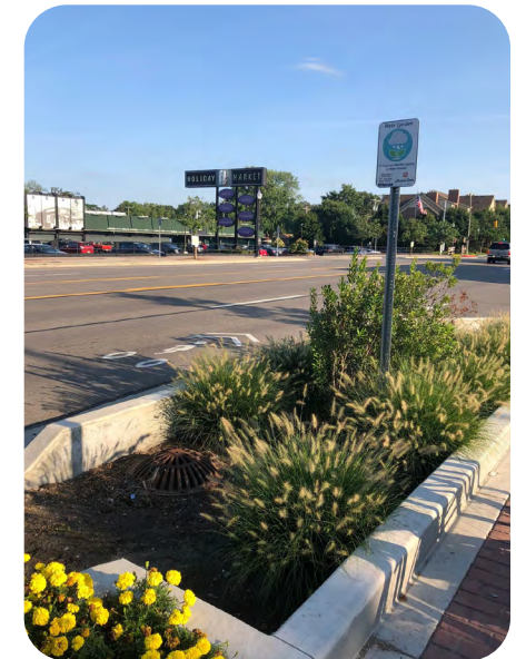
This rain garden is integrated into the South Main Street streetscape in Royal Oak. It allows stormwater runoff to enter and infiltrate under normal conditions, while a catch basin structure provides additional capacity during larger rain events.
