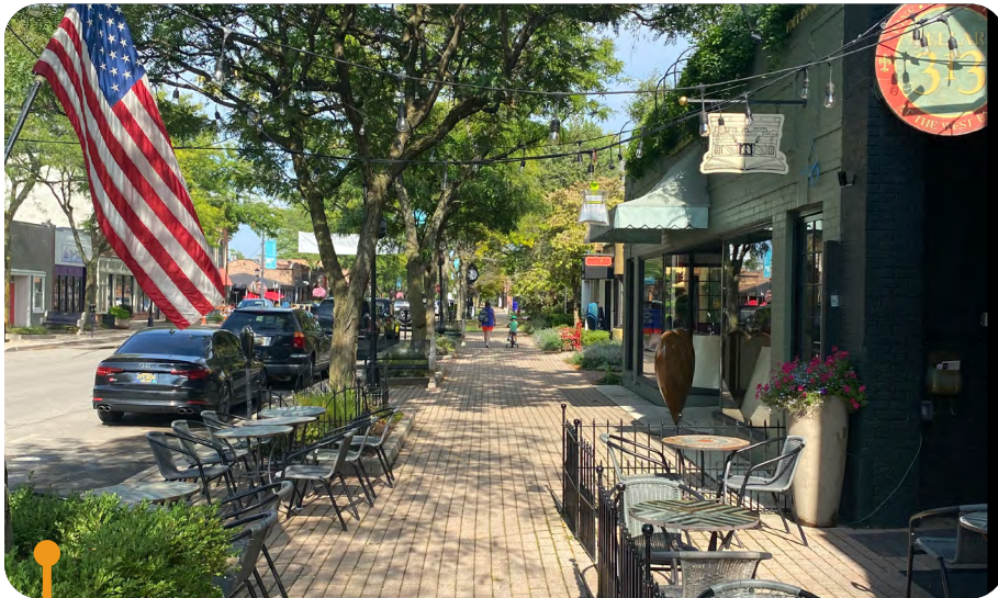
Well-planned street trees enhance the pedestrian experience by providing shade and creating a natural buffer between visitors and traffic.
