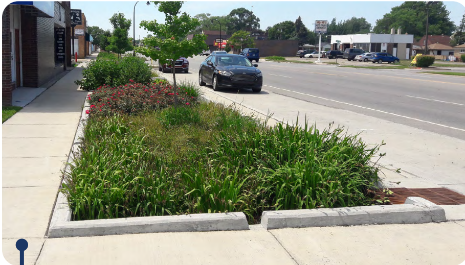
Sidewalk green infrastructure bioretention in Allen Park captures and infiltrates stormwater from surrounding impervious surfaces. It also helps with traffic calming and serves as a buffer for pedestrians.
