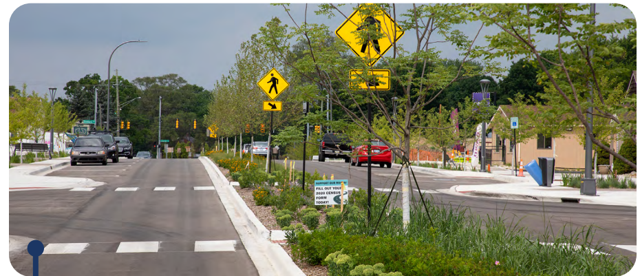
Pedestrian refuge island in the Brooklands District in Rochester Hills gives a place to stop when crossing the street and is designed to capture stormwater.
