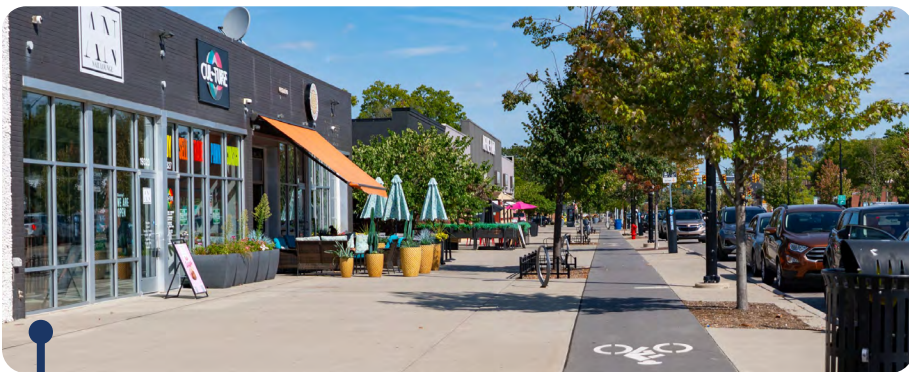
The Livernois–McNichols Main Street in Detroit was recently redesigned with large sidewalks, giving ample space for outdoor dining, a clear pedestrian path, a wide planter/furniture zone, and separated bike lanes.
