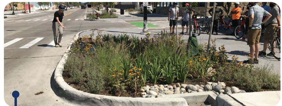
Curb bump out in the Livernois-McNichols Main Street in Detroit reduces the crossing distance for pedestrians from four lanes to two lanes, while also acting as a reservoir for stormwater
