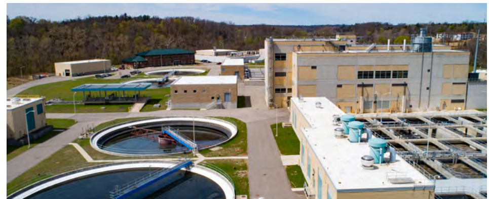
Wastewater treatment plant in the City of Ann Arbor
